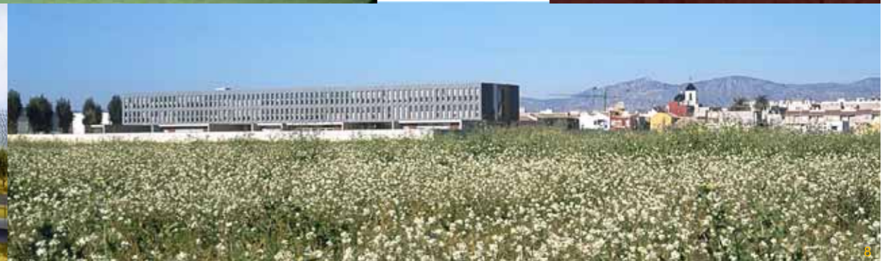
Secondary school Dolores, Alicante. (1994-2004) photo 8
